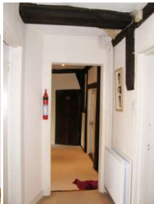
First floor corridor
